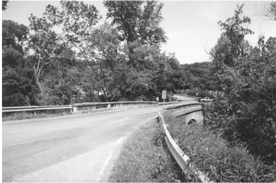
Figure 5–6. Tollgate Ridge Road bridge over Great Tonoloway Creek. Looking west.
