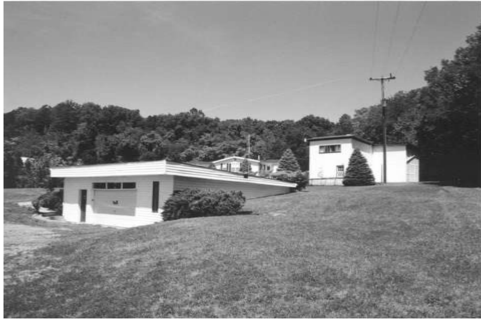
Figure 5-8. Hancock Drive-in concession stand and projection booth. Note berms in foreground and new house in background.
