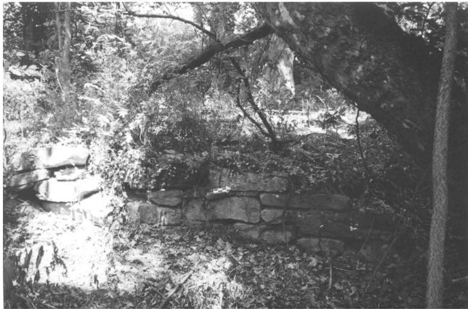
Figure 5–23. Stone revetment of the headrace.
