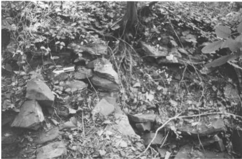
Figure 5-31. Top of north wall in gully, looking east.
