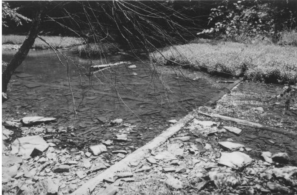
Figure 5–18. Timber cribbing, Timber #s 1, 4, and 5.
