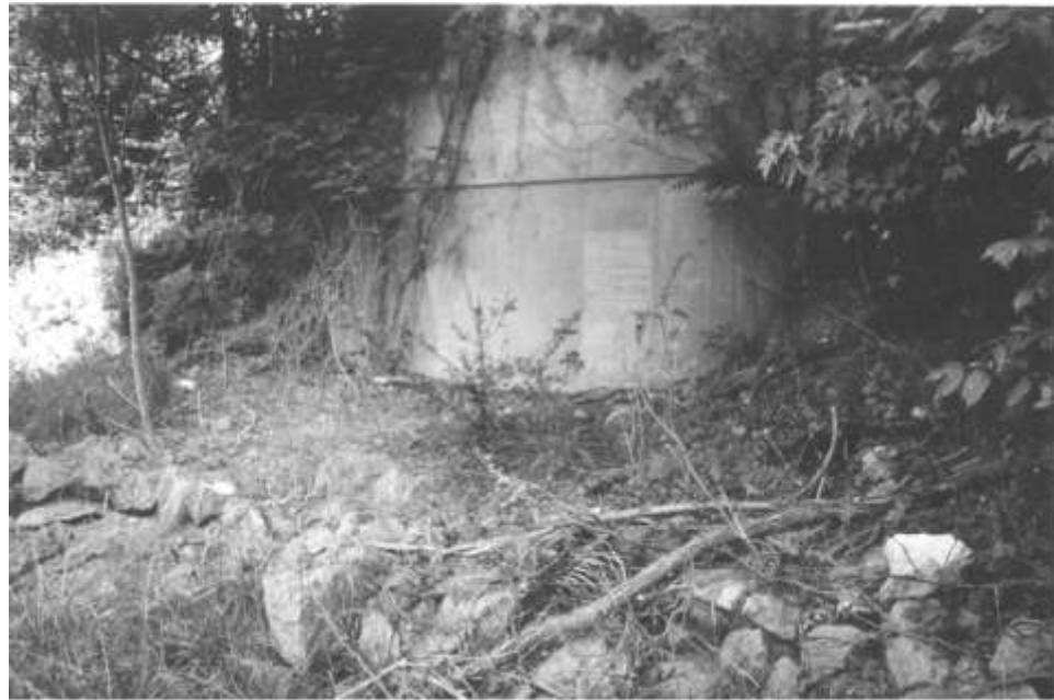
Figure 5–33. Northeast bridge pier and stone revetment, looking northwest.
