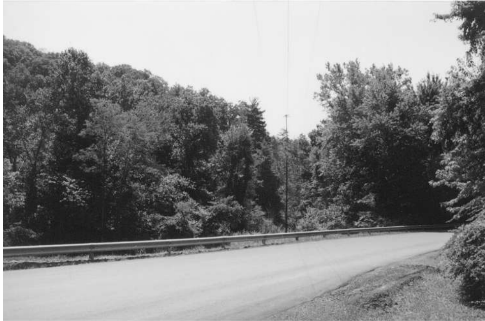
Figure 5-11. Realigned portion of Rayloc Road. Looking south across creek. Note new utility line.
