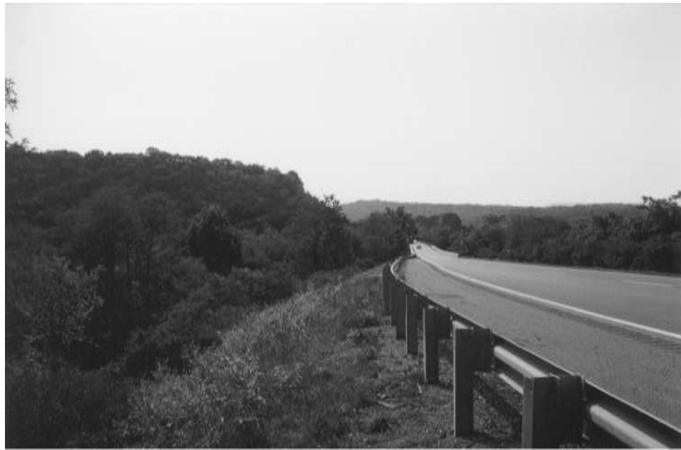
Figure 5–3. North end of project area looking southeast to bridge.
