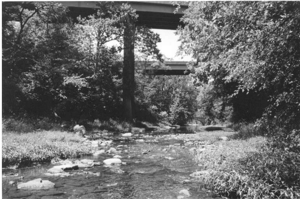
Figure 5–17. Creek from dam remnant to I-70 bridge.
