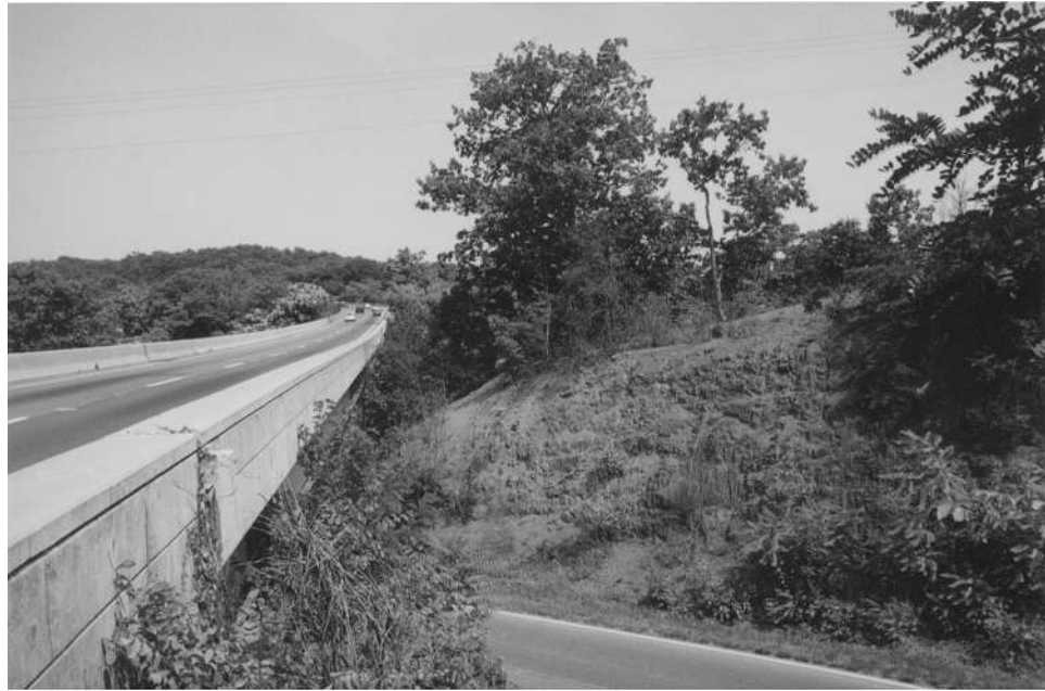
Figure 5-4. I-70 overpass and Timber Ridge Road.
