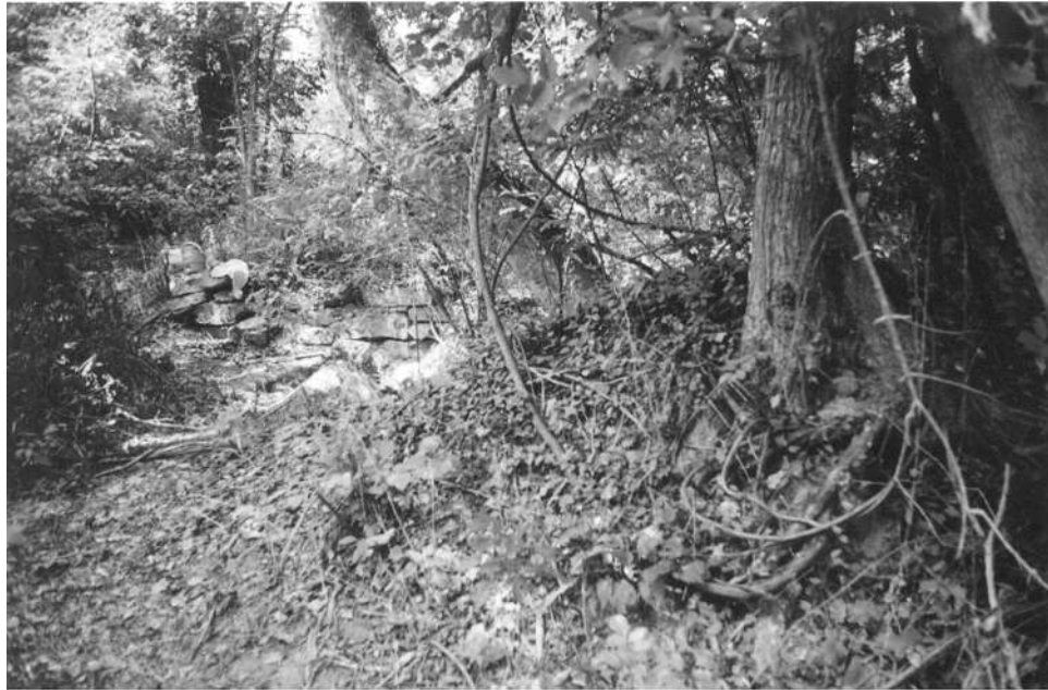
Figure 5–22. Earthen dam remnant with protruding tree.
