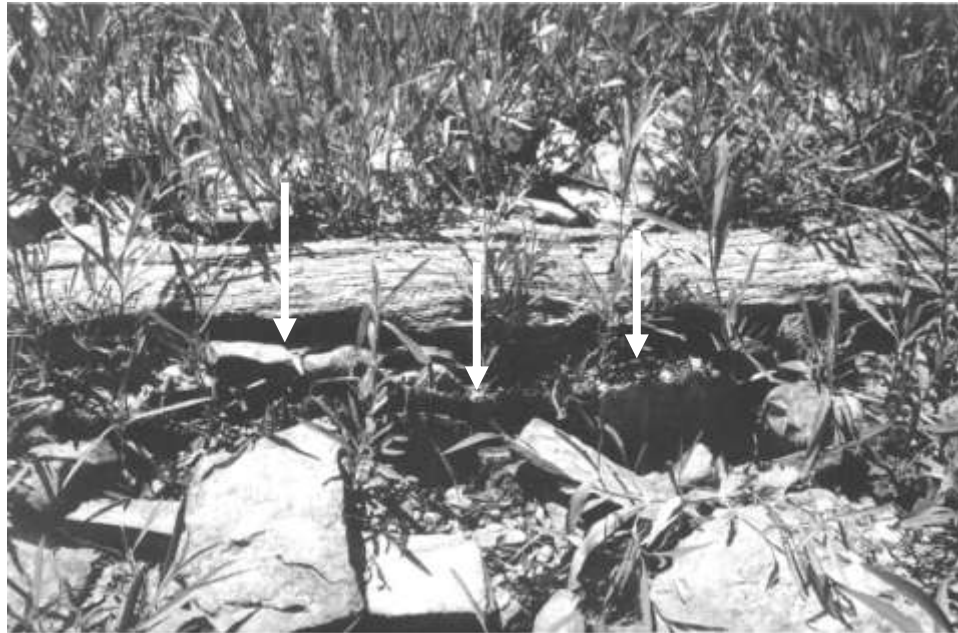
Figure 5–19. Exposed cribbing and vertical boards, Timber #8.
