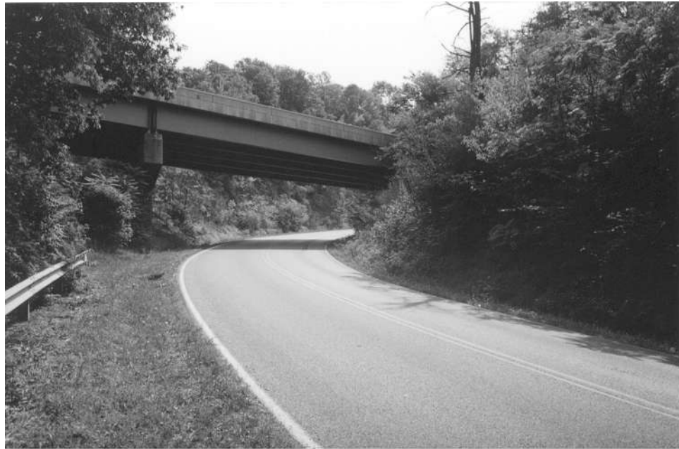
Figure 5-5. Timber Ridge Road, looking east, and I-70 overpass.
