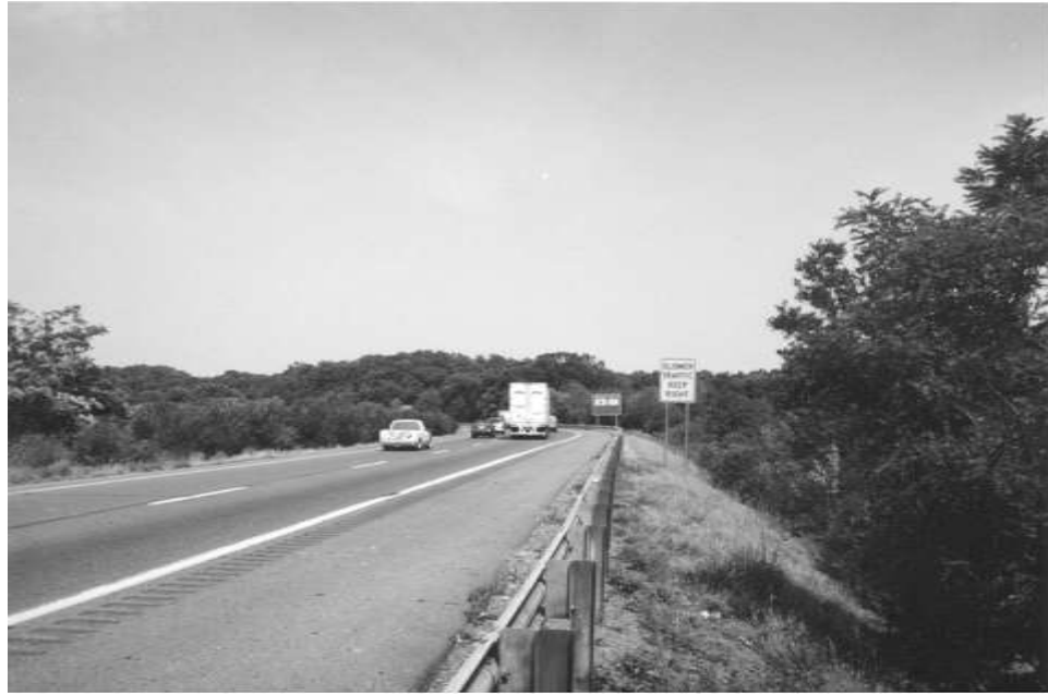
Figure 5–2. North end of project area, westbound lanes.
