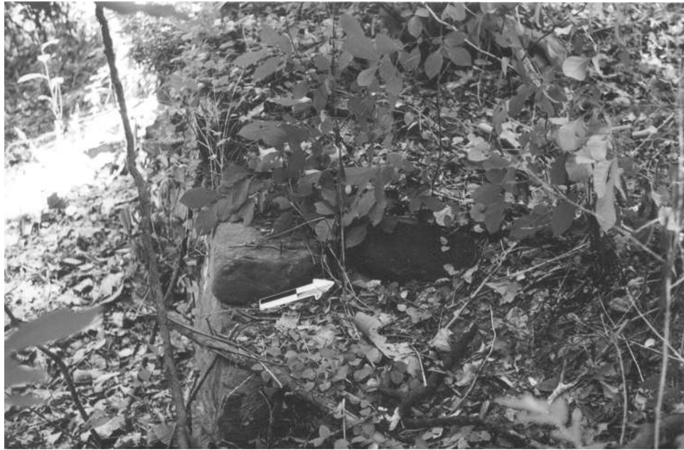
Figure 5-26. Top of headrace retaining wall, looking west.
