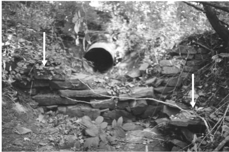
Figure 5–29. Culvert, gully, and walls. White arrows indicate walls.
