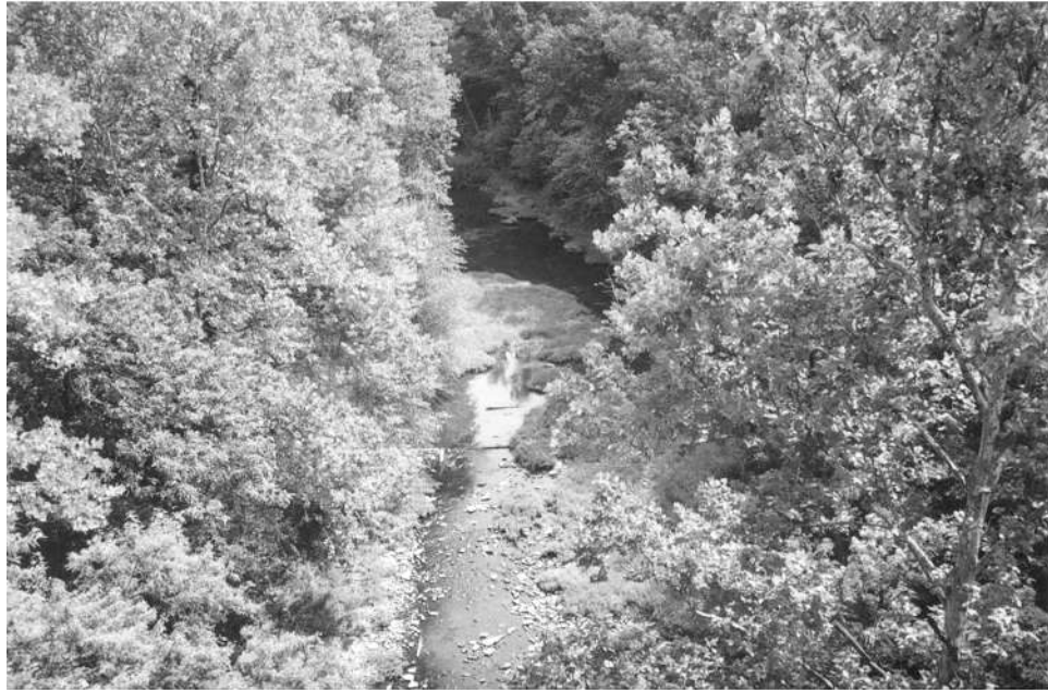
Figure 5–16. Dam remnant in creek, middle ground.
